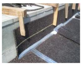
Vertical sections can be fixed using temporary mechanical devices (e.g. clamps, etc.). Ensure that no metal fixings are left in place that can cause sound bridging. The bonding of the side areas is over entire surface.
